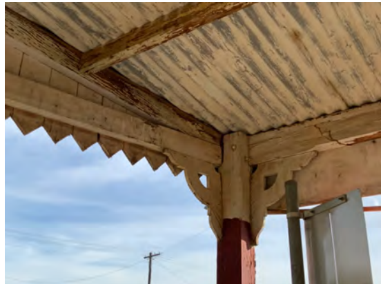
Figure 8: Detail of the front awning, showing decorative timber brackets and timber valance.
