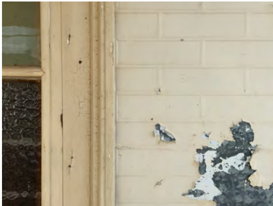
Figure 7: View of the front masonry pattern tin cladding.
