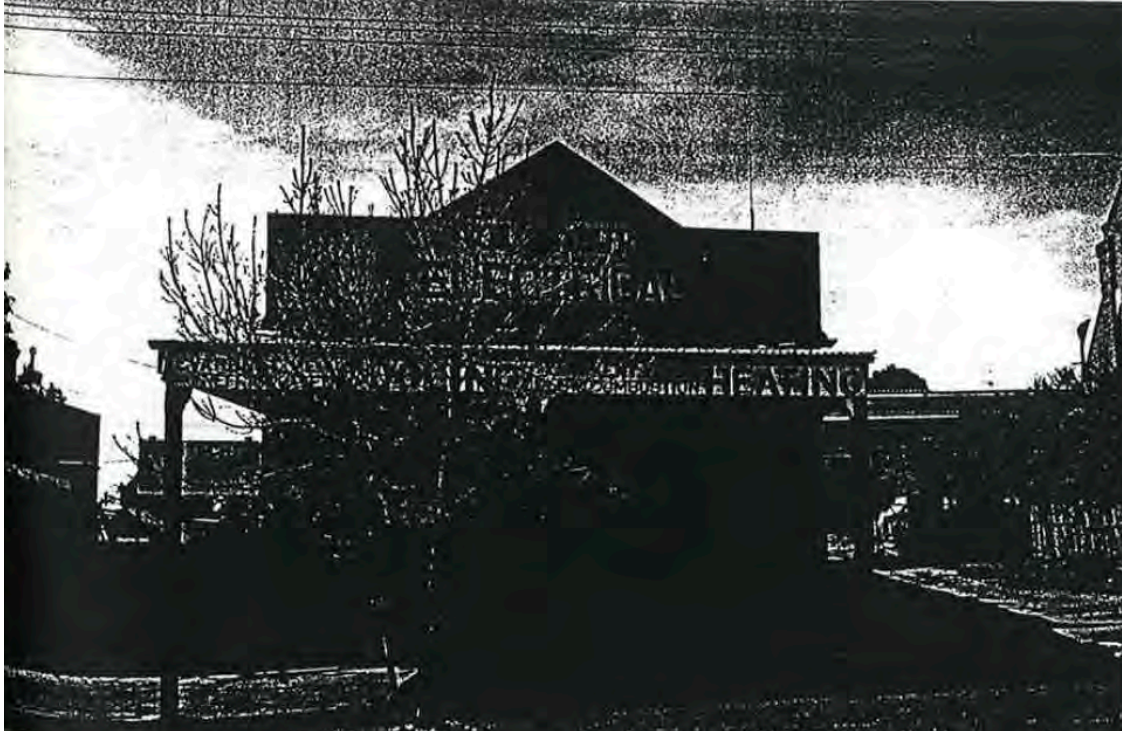
Figure 32: View of the subject site in 1992. Despite the poor quality of the image, the photo evidences the extant overall form of the building as viewed from Forbes Street. It shows the existence of the skillion roofed awning off the southern side elevation and the various signage applied to the gabled façade above the awning and fascia signage to the awning itself.
