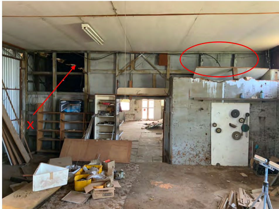
Figure 34: View of the building facing towards Forbes Street, showing the areas of visible deterioration. The charred timber framing (painted silver) is shown. Note: due to safety concerns, access to the roof void was not obtained, but observations made from standing at the location marked 'X' and facing in the direction of the arrow as shown.
