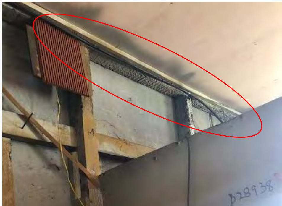
Figure 35: Evidence of some of the more visible fire damage to the building.
